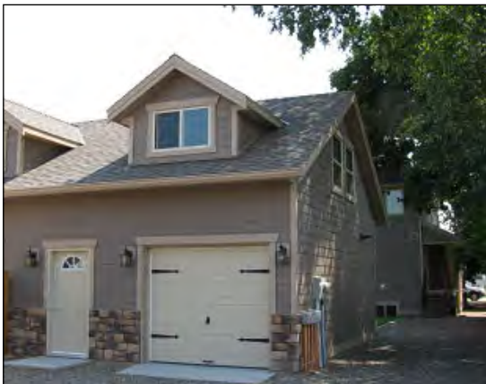
Unit built above garage
