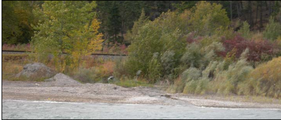
Segment 7. Marion Creek flow entering into the lake through a culvert under the railway. Photo: Porto Sept 2007.
