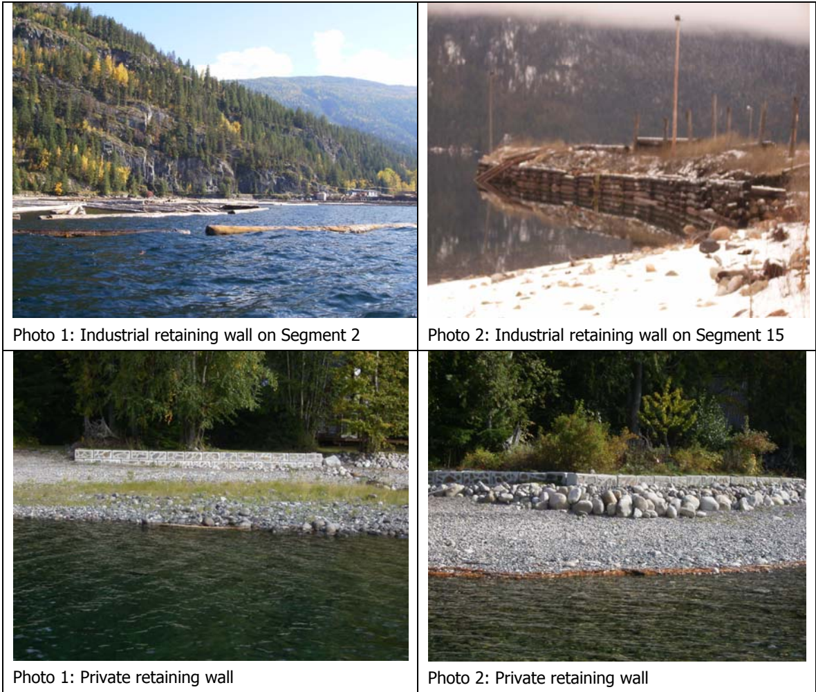
Figure 12: Industrial and private retaining walls along Slocan Lake foreshore
