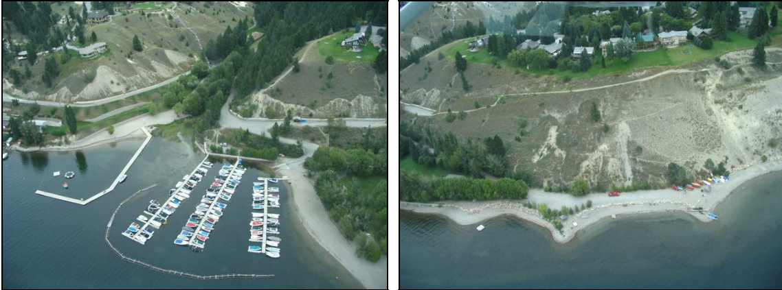
Figure 16. North end of Segment 22 showing the public park along the north side of Holland Creek, and the Timber Ridge marina and beach private recreational properties.
