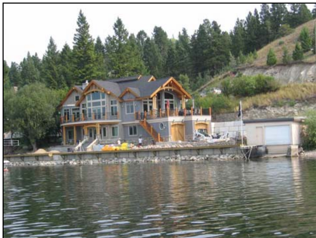
Figure 20. Foreshore modifications include removal of riparian vegetation, construction of retaining walls, docks, and boat houses.
