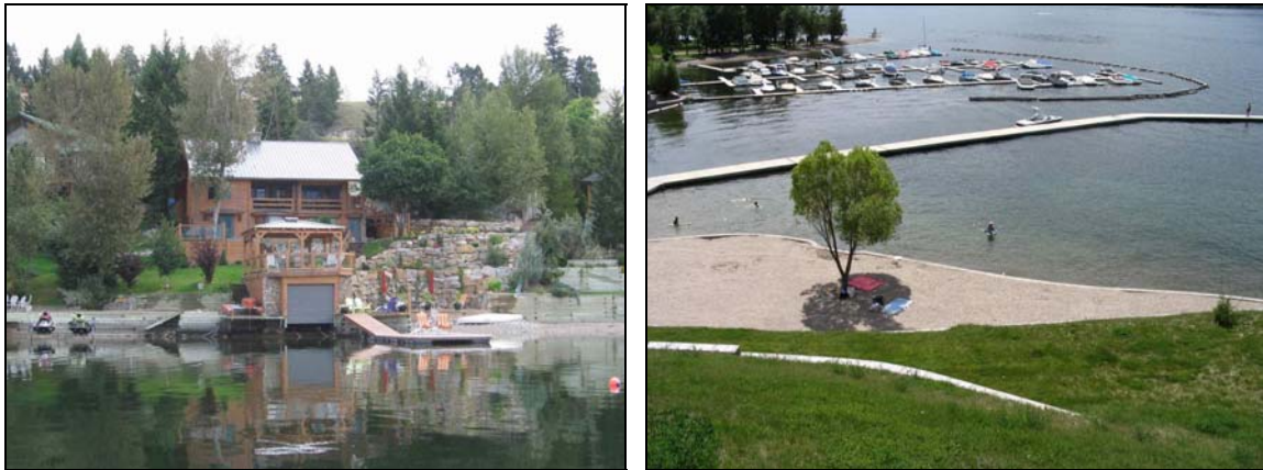
Figure 4. Examples of foreshore modifications along Windermere Lake, including boathouse, dock, retaining wall (left); and marina, dock and retaining wall (right, [photo provided by Wildsight]).
