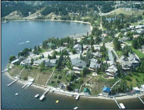
Segment 16 (residential area in foreground)
