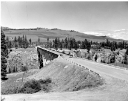
Rock Creek Bridge BCAR i-21953
