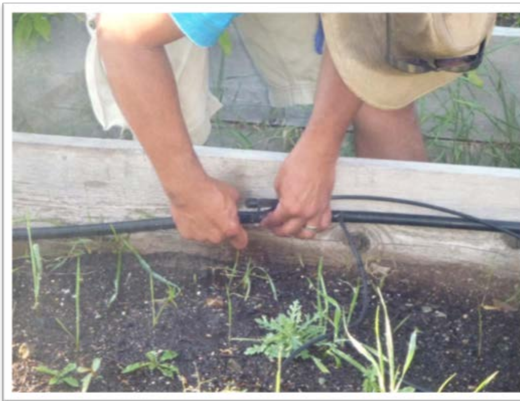
Figure 5. Drip irrigation being installed at the Kettle River Community Garden.
