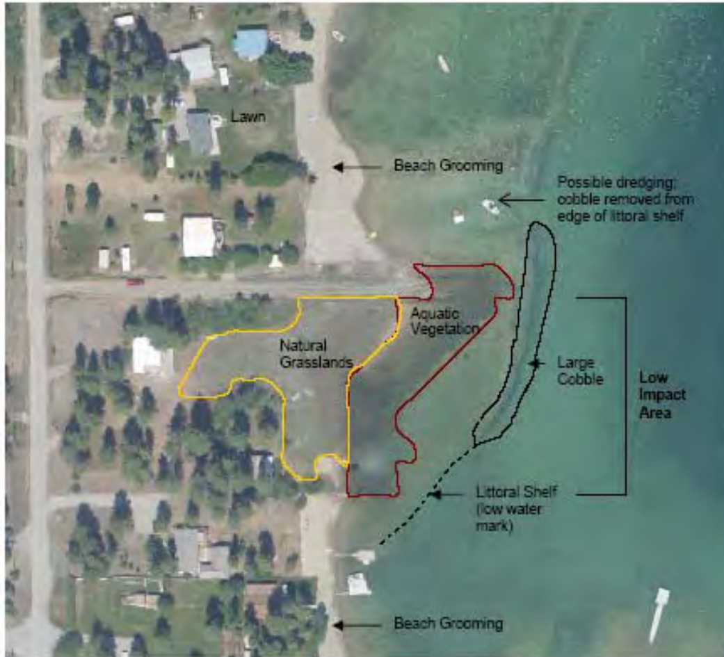
Figure 20. Overview of properties along Segment 3, showing area where the natural shoreline features were kept intact (low impact area) against adjacent properties where development has substantially altered the shoreline.
