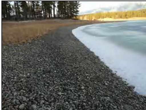
Figure 11. Cobble shoreline following the base of the Vegetated shore type of Segment 6.
