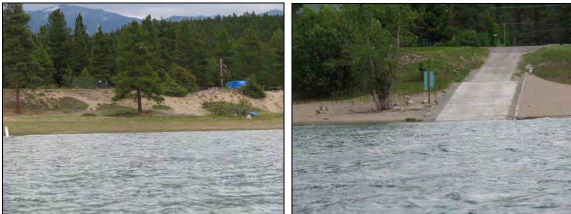
Segment 9: An example location where grass/herb vegetation has been maintained along the shoreline and of houses situated up on a bench (left) and boat launch/groyne structure at end of the segment (right). Photo: Holmes, June 2008.
