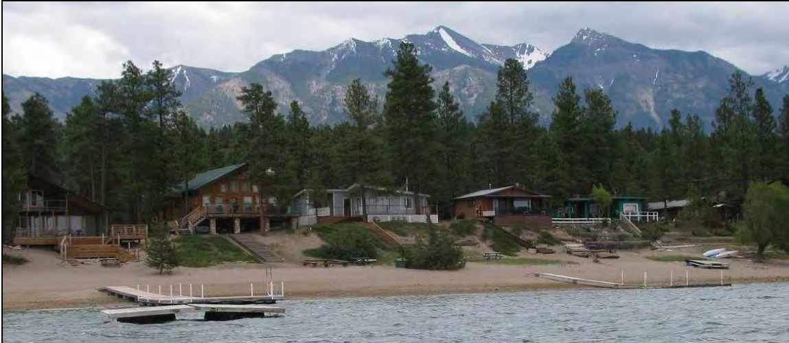
Figure 25. High Level of Impact example (Segment W1), showing how development has impacted all of the shoreline. Photo: Holmes July, 2008.
