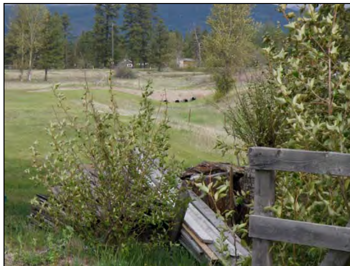
Figure 4. Swale and culverts beneath private roadway to direct high flows between Cameron Pond and Wasa Lake. Photo: McPherson, May 2010.
