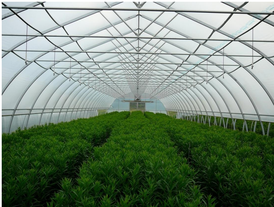
Figure 5. View of the growing space and internal frame of a 30' wide Gothic style greenhouse manufactured by B&W Greenhouse.
